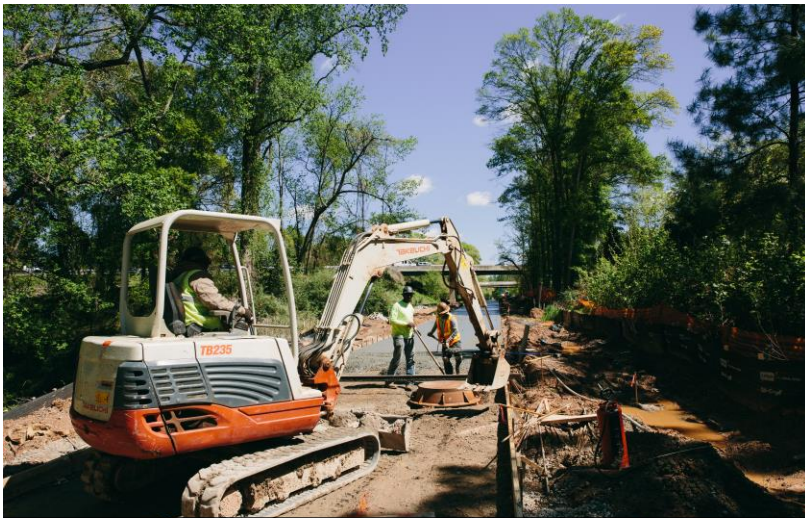
Westside Trail Under Construction
